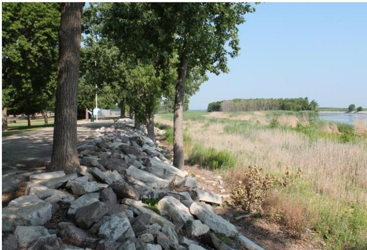
**Figure 10.** Shoreline erosion control feature at Bay Beach.
