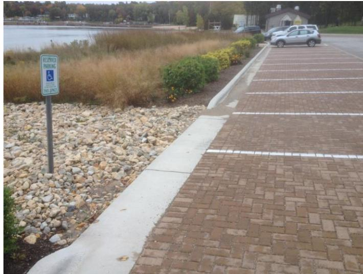
**Figure 7:** Porous pavement and vegetated swale at a Door County beach parking lot.
