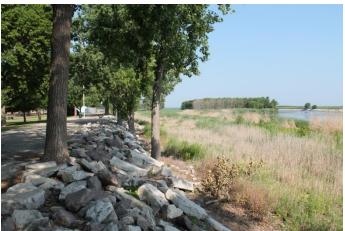
Figure 8. Shoreline erosion control feature at Bay Beach.
