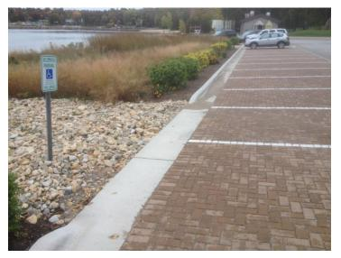
Figure 9: Porous pavement and vegetated swale at a Door County beach parking lot.
