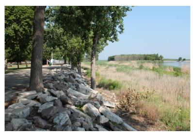
Figure 10. Shoreline erosion control feature at Bay Beach.
