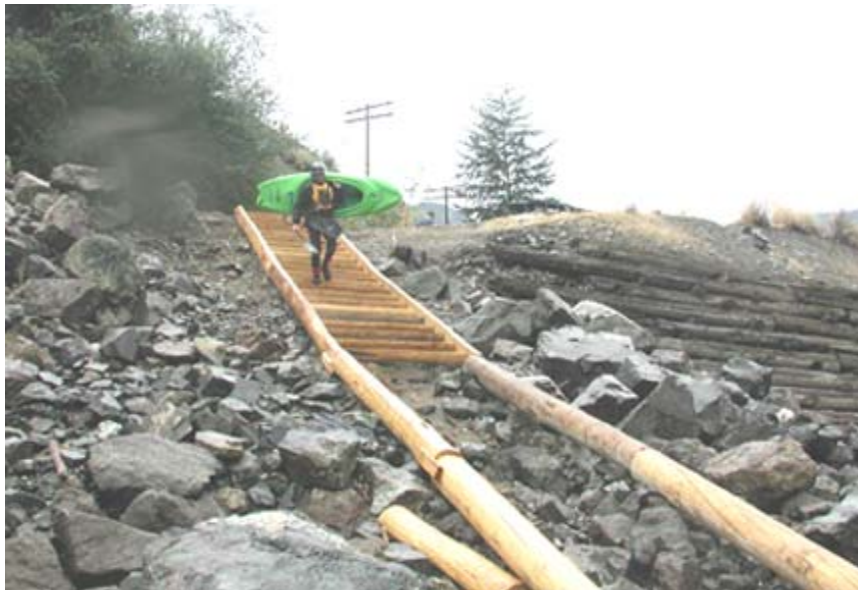
Photo 9E: Rounded timbers serve as staircase for paddlers
