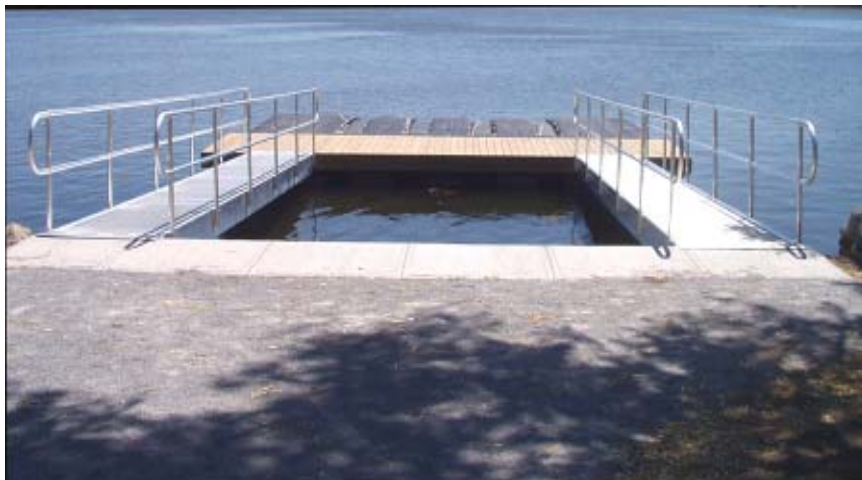
Photo 5A: Floating launch provides access to Hudson River at varying water levels
