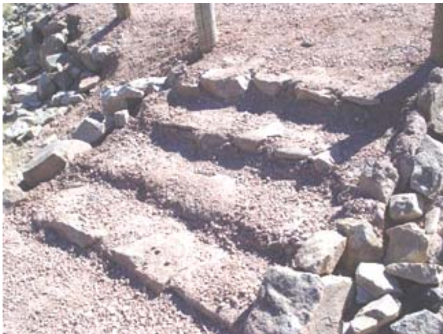
Photo 9H: Rock staircase reinforced with rip-rap form a simple staircase to launch area
