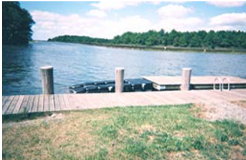
Photo 5D: Floating launch attached to bulkheads can be accessed from the shore by a ladder
