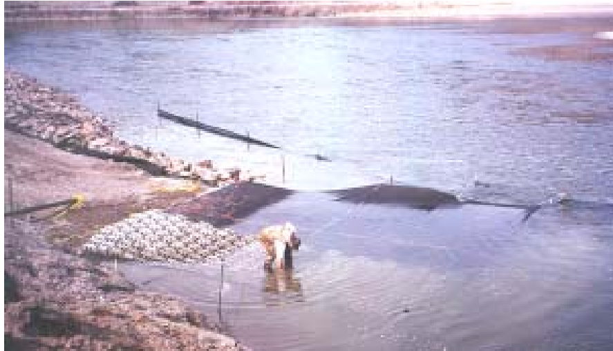
Photo 8J: Concrete mats are installed individually
