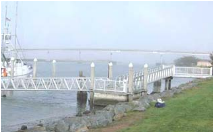
Photos 3A, 3B: An approach ramp, with a fixed slope of 8.33%, connects floating launch to the shore
