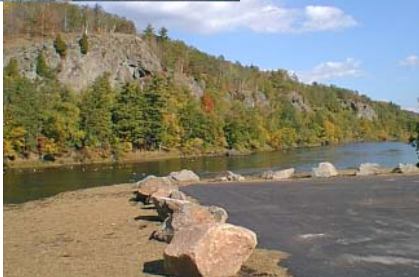
Photo 10D: Little Quinnessec Falls launch area, reinforced with fractured rock riprap
